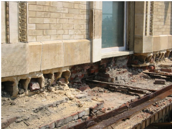
Figure 25. Severe corrosion of cornice support steel. Also note back up masonry included terra cotta in compression.
