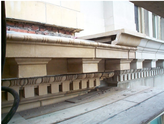
Figure 39. New GFRC modillion course and original terra cotta egg and art / dentil course
