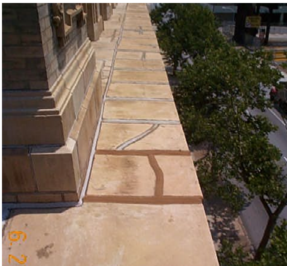
Figure 4. Previous sealant application at cornice cracks
