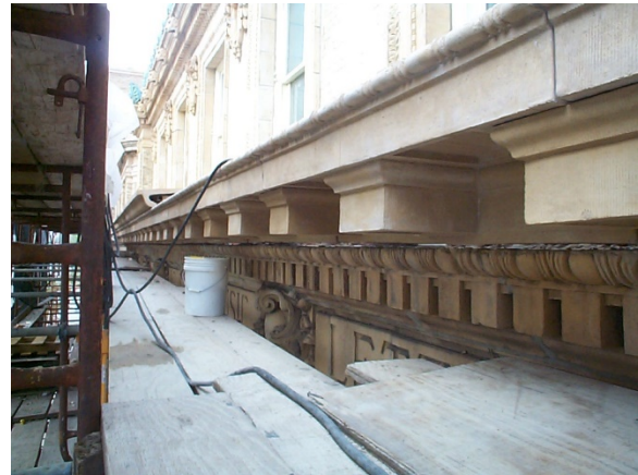
Figure 40. New GFRC modillion course and original terra cotta egg and art / dentil course
