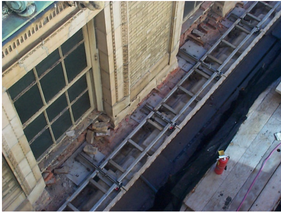
Figure 31. New stainless steel support frame in place
