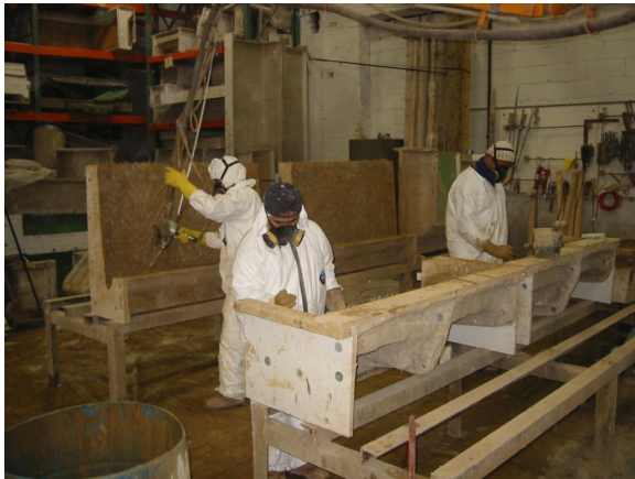
Figure 15. Hand spray fabrication of GFRC
