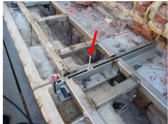
Figure 30. Back-to-back angle outriggers and 'J'-hooks to support suspended modillions below.
