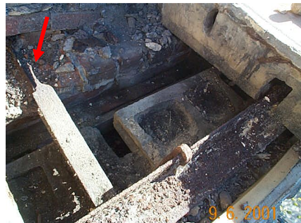
Figure 8. Severely corroded outrigger beam. Top flange is gone.
