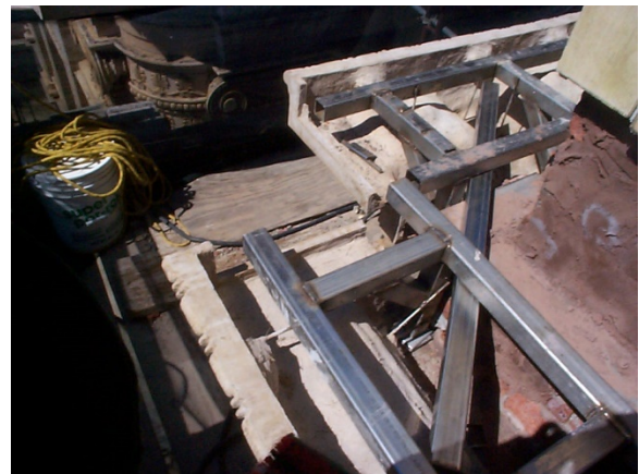
Figure 34. Corner framing partially complete
