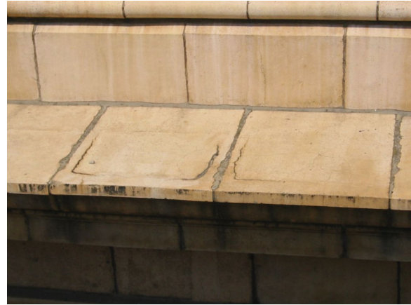
Figure 3. Cracks at shell/rib
