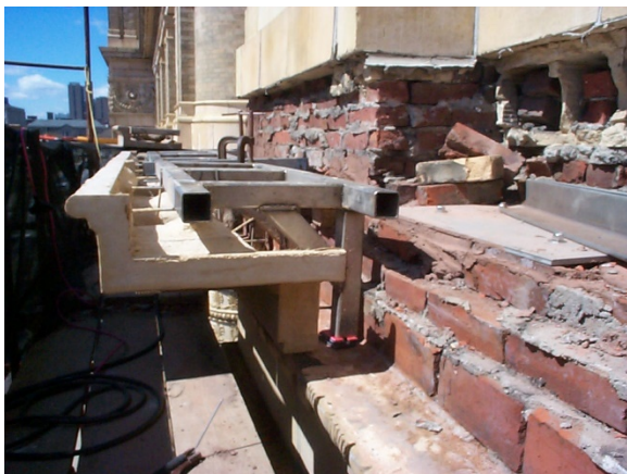
Figure 35. Cantilevers embedded, lower units installed and back up masonry repaired.
