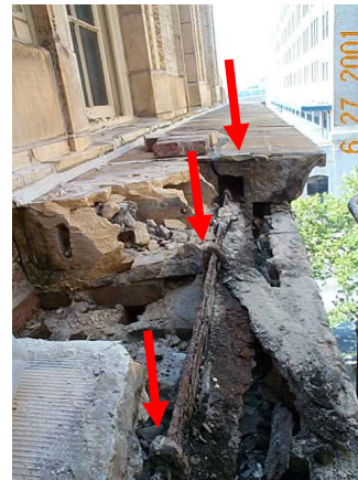
Figure 6. Severely corroded back-to-back steel angles aligning with cracks in terra cotta cornice. Outer portion of the cornice is a potential fall hazard.
