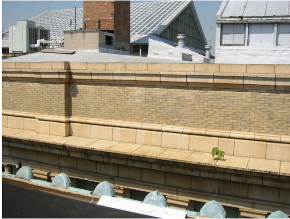
Figure 2. Vegetation growth from mortar joint
