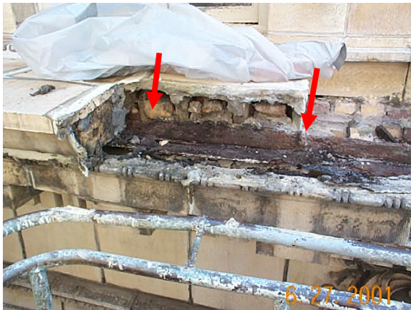
Figure 5. Severely corroded back-to-back steel angles. Arrows point to ‘J’-hook modillion hanger.
