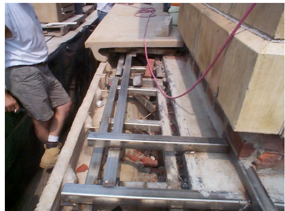
Figure 36. Capstone installation
