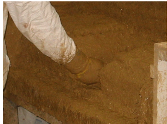
Figure 18. Back rolling fiber consolidation
