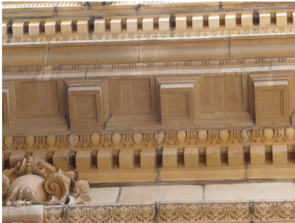
Figure 45. GFRC modillion course on top of original terra cotta dentils
