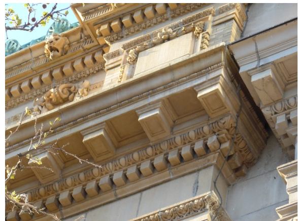
Figure 48. Close up. Note, modillion course and cornice above is 16-year old GFRC, all other masonry is historic terra cotta.
