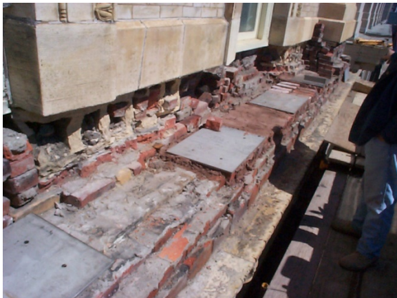
Figure 29. Cantilever base plates installed
