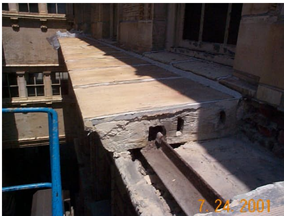
Figure 10. Some locations the steel had not corroded severely and the terra cotta was in good condition. These were used for models
