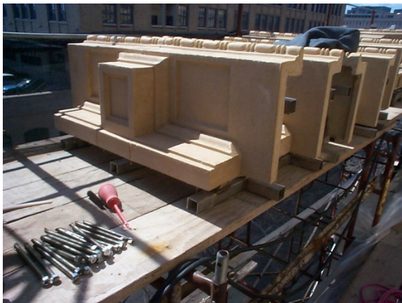
Figure 33. Lower course units. Note these were originally 5 separate units.
