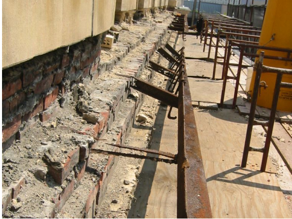
Figure 27. Outriggers failed under their own weight.
