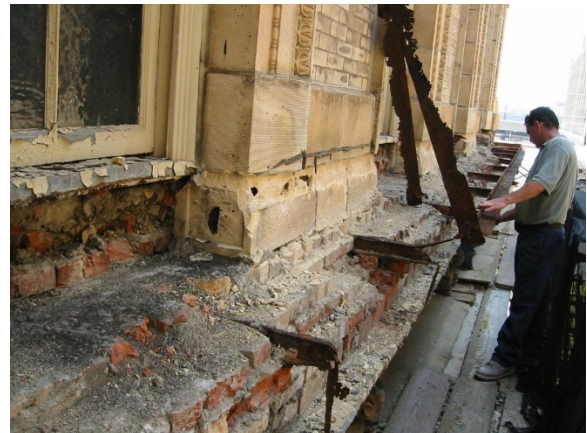
Figure 26. Failed outrigger beams and terra cotta units at base of pier in compression.
