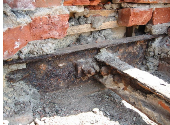
Figure 28. Severe corrosion at joint with embedded façade beam and outrigger
