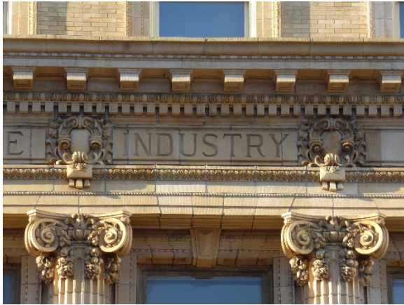
Figure 44. 11-year old GFRC cornice and modillions integrated into historic terra cotta.
