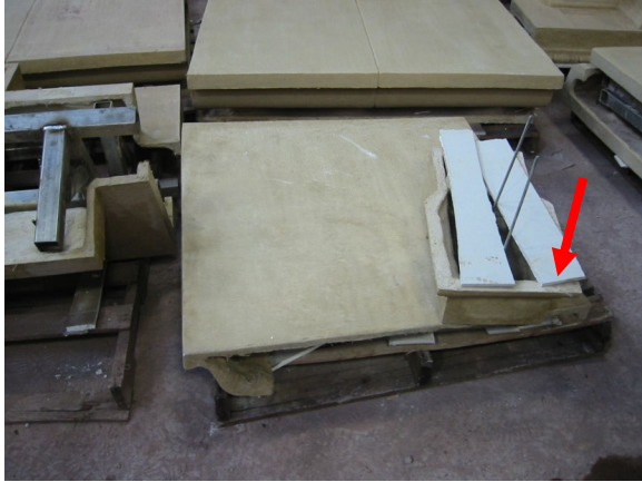
Figure 23. Top course with shoulder to integrate with existing terra cotta window surround.
