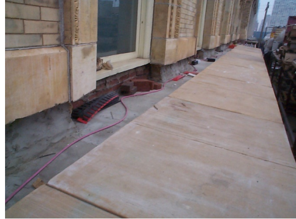
Figure 38. Back up masonry repaired and parged
